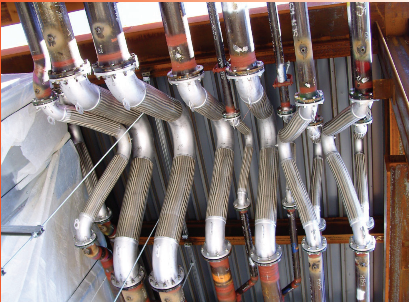
VERTICAL VFL INSTALLATION (Apex Near Ceiling)
